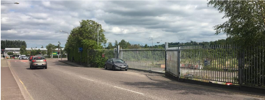
Plate 12.1 Access gate to subject site on Tramore road
